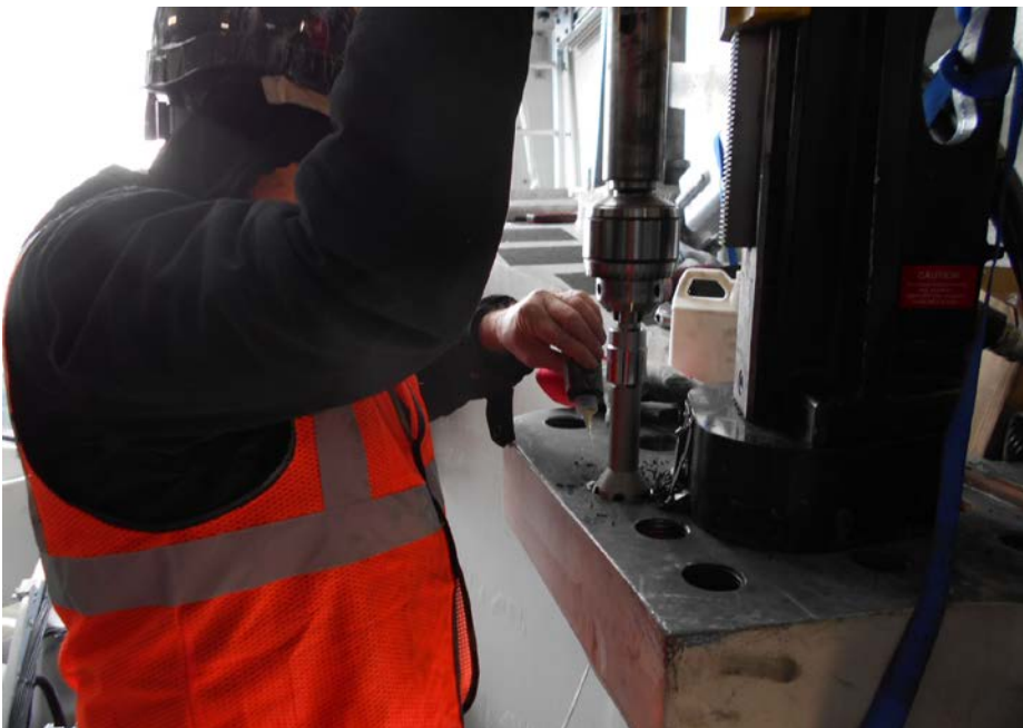
Wind turbine repair of damaged threads by QuantiServ
